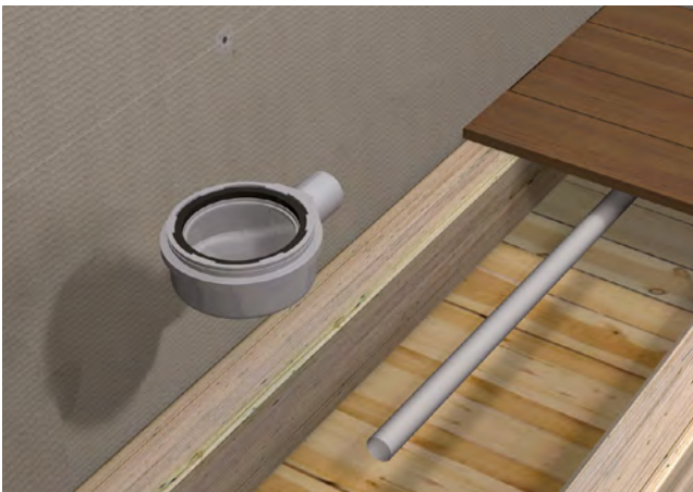
2. Install the waste ensuring adequate run off.
