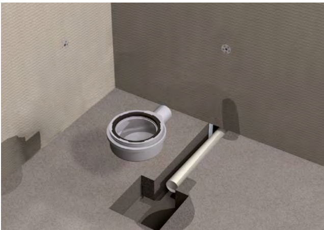
2. Fit the horizontal waste into position within the concrete floor.
